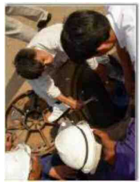
Water supply project at Phnom Penh
