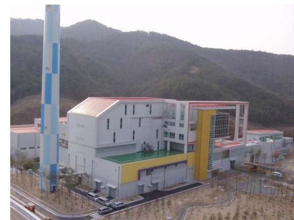
Gumi Plant, South Korea 100 t/24h x 2unit (2010)
